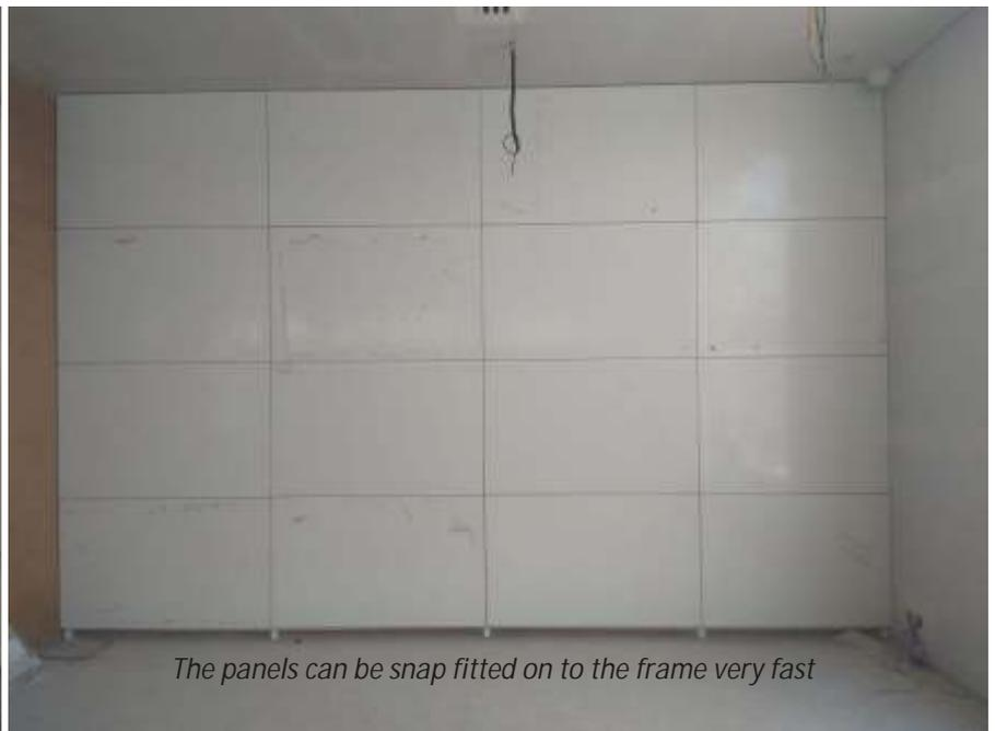
*The panels can be snap fitted on to the frame very fast*
