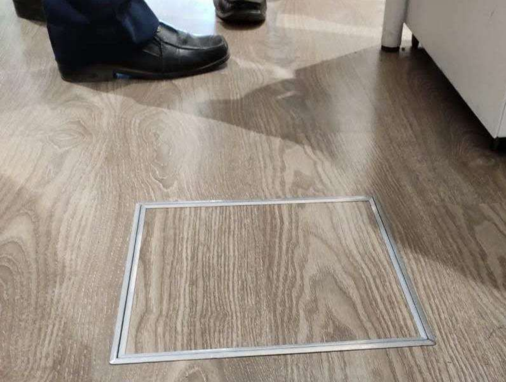
JB22 / 23 Floor Junction Box, with wood plank, carpet and tile embedded in lid
