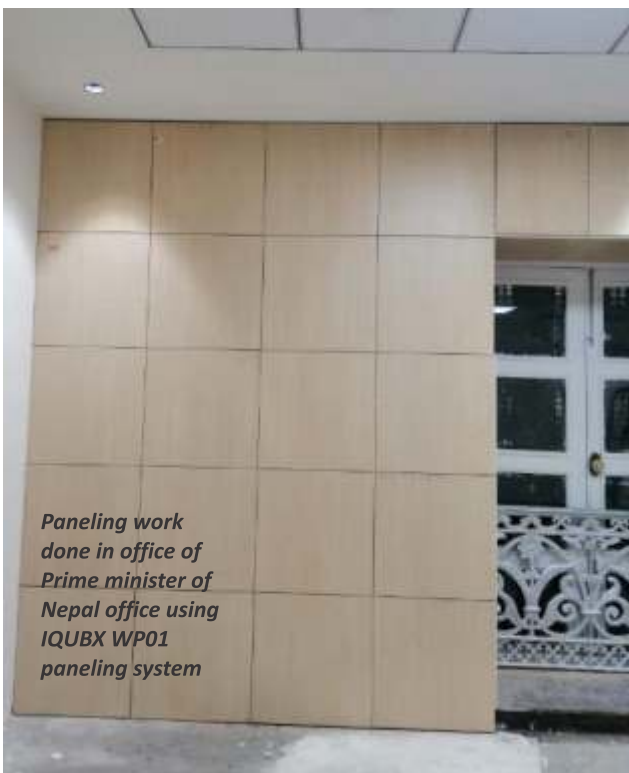
The panels can be snap fitted on to the frame very fast
