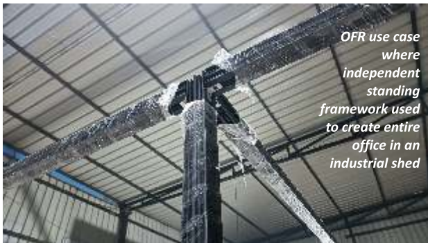
Main frame made of 50 x 50 IQUBX aluminium green certified proprietary section of open frame rack system.
