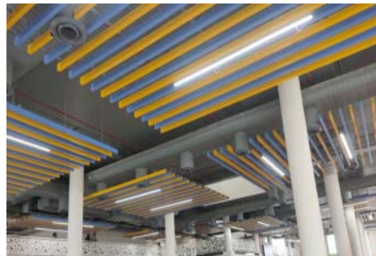
Conversion of standard extrusion tubes into a baffle with proprietary clips is possible
